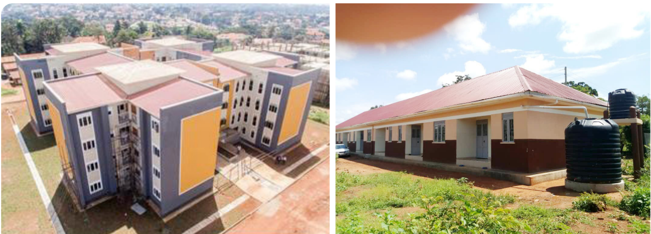
Picture 2: Staff Accommodation blocks under construction at Naguru and Budaka.
